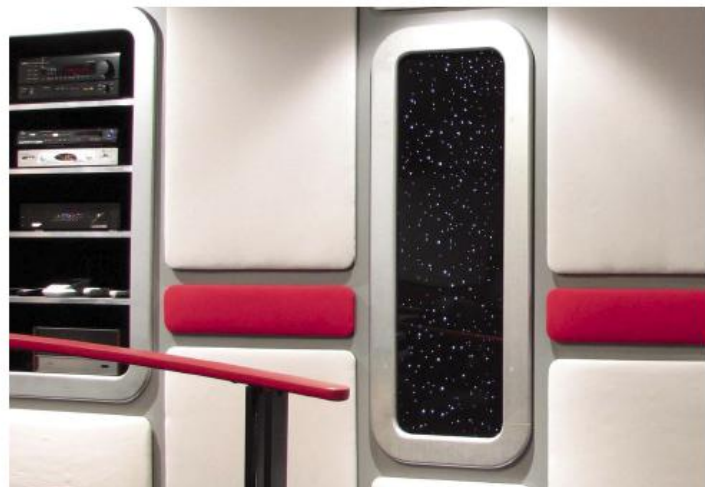
SPACE ISSUES The rack of components is accessible from a closet on the other side of the wall, and a cleverly crafted view port is set between acoustic treatments.
